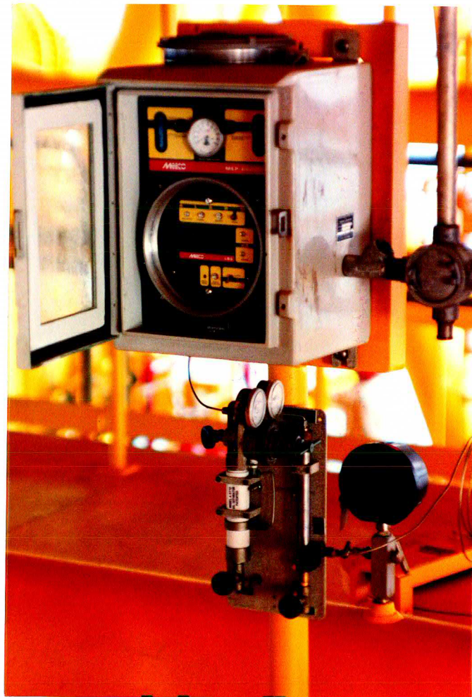
MEECO MEP-BRAVO Moisture Analyzer Used in a Gulf offshore application.
